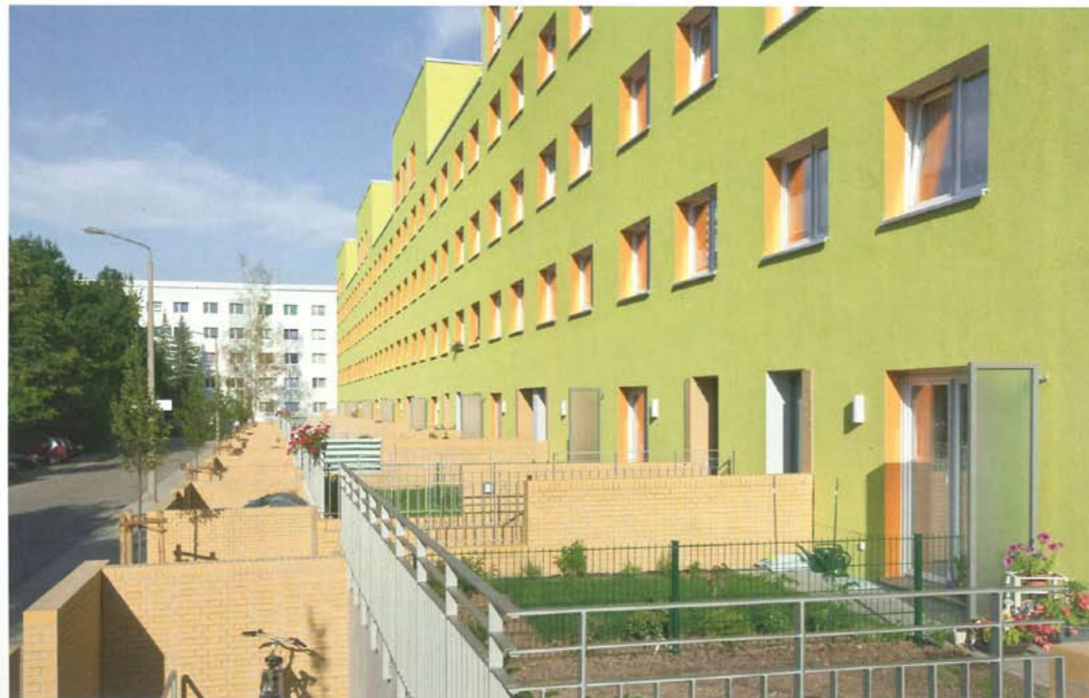
↓ Street side with new plinth
