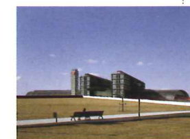
48. Berlin Central Station gmp – von Gerkan, Marg and Partners Architects Berlin, 2006
