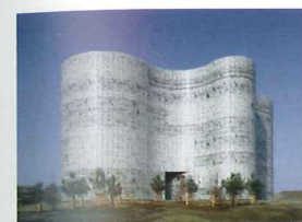
31. IKMZ BTU Cottbus, Information, Communications and Media Centre Herzog & de Meuron Cottbus, 2004
