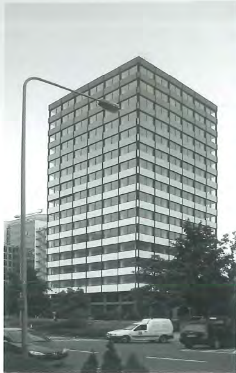
Bürohochhaus, Zustand Mai 2007 Office highrise, condition in May 2007
